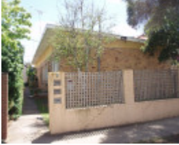
7 Verner St, Geelong South
