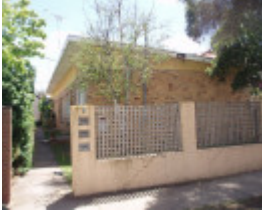
7 Verner St, Geelong South
