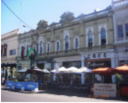
'Salisbury Buildings', Hobsons Bay Heritage Study 2006
