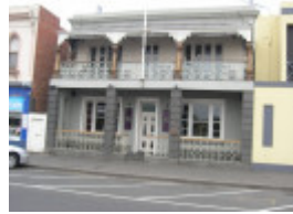
Wilkins House / Claredon Hotel (former), Hobsons Bay Heritage Study 2006
