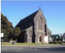
Holy Trinity Church of England Complex, Hobsons Bay Heritage Study 2006
