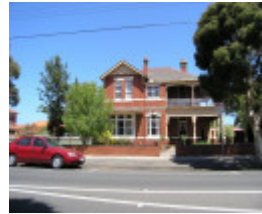
St Joseph's Roman Catholic Convent and Presbytery, Hobsons Bay Heritage Study 2006
