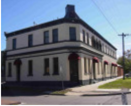
Newport Coffee Palace (former), Hobsons Bay Heritage Study 2006
