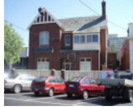
Maclean Residence and Surgery (former), Hobsons Bay Heritage Study 2006
