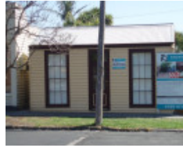
Shop and Residence (former) at 28 Parker Street WILLIAMSTOWN, Hobsons Bay Heritage Study 2006
