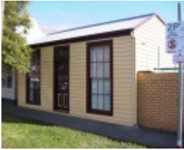
Shop and Residence (former) at 28 Parker Street WILLIAMSTOWN, Hobsons Bay Heritage Study 2006
