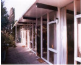
House at 19 Pearson Street WILLIAMSTOWN, Hobsons Bay Heritage Study 2006
