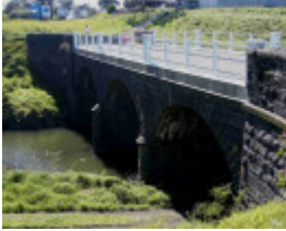
Bluestone Bridge over Kororoit Creek Road, Hobsons Bay Heritage Study 2006
