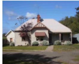
Truganina Explosives Magazine Complex (former) and trees, Hobsons Bay Heritage Study 2006
