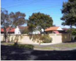
House at 2 Seaview Crescent SEAHOLME, Hobsons Bay Heritage Study 2006
