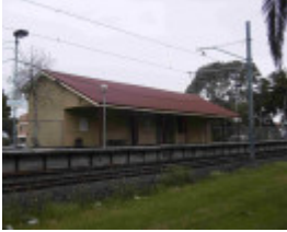
Seaholme Railway Station Complex and trees, Hobsons Bay Heritage Study 2006
