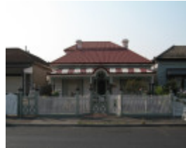
Alcroft at 13 Station Road, Hobsons Bay Heritage Study 2006
