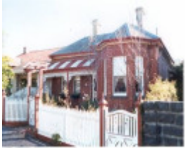
House at 8 Stevedore Street WILLIAMSTOWN, Hobsons Bay Heritage Study 2006
