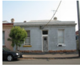
Shops (former) and Residences at 46-48 Stevedore Street WILLIAMSTOWN, Hobsons Bay Heritage Study 2006 - No 46
