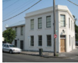
Napier Hotel (former), Hobsons Bay Heritage Study 2006
