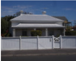
House at 12 The Strand WILLIAMSTOWN, Hobsons Bay Heritage Study 2006
