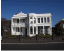
House at 14 The Strand WILLIAMSTOWN, Hobsons Bay Heritage Study 2006
