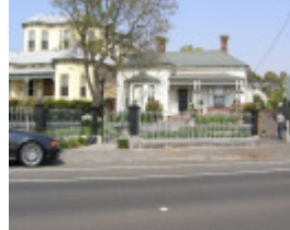
House at 75 The Strand NEWPORT, Hobsons Bay Heritage Study 2006
