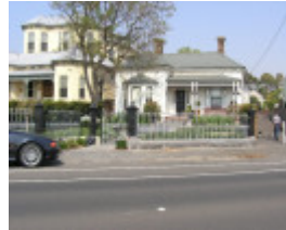
House at 75 The Strand NEWPORT, Hobsons Bay Heritage Study 2006
