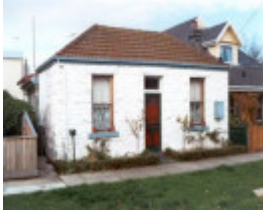
House at 97 Thompson Street WILLIAMSTOWN, Hobsons Bay Heritage Study 2006
