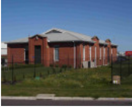
Commonwealth Oil Refinery Complex (Former), Hobsons Bay Heritage Study 2006
