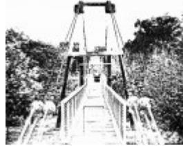
City of Kew Urban Conservation Study 1988 - Footbridge
