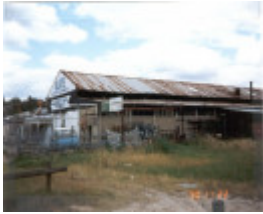
22351 Shed (Aust Slate Co) - 402 Doncaster Road, Balwyn North
