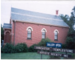
22383 Shire Offices (former) - 673 Doncaster Road, Doncaster (1)
