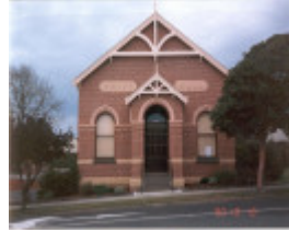
22383 Shire Offices (former) - 673 Doncaster Road, Donacster (2)
