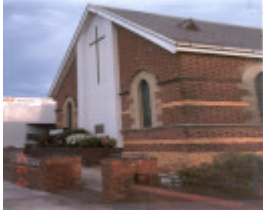
22384 Doncaster Church of Christ - 680 Doncaster Road, Doncaster (1)
