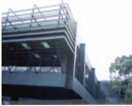
22387 Manningham City Council Municipal Offices (fmr Doncaster & Templestowe Council) - 699 Doncaster Road, Doncaster (1)
