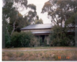
22398 House - 88-90 George Street, Doncaster (2)
