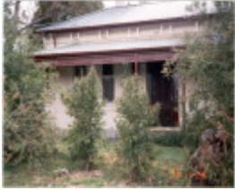
22398 House - 88-90 George Street, Doncaster
