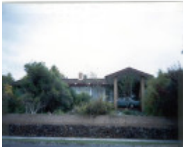
22406 L. Crooks House - 18 Tower Street, Doncaster
