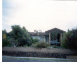
22406 L. Crooks House - 18 Tower Street, Doncaster (2)
