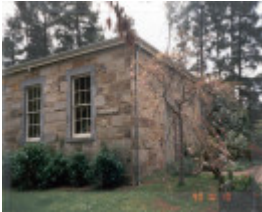
22410 Schramms Cottage - 62-78 Victoria Street, Doncaster (1)
