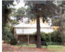
22410 Schramms Cottage - 62-78 Victoria Street, Doncaster (2)
