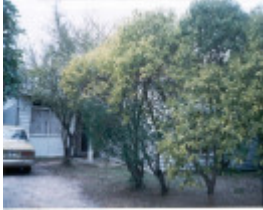
22421 House - 108 Whittens Lane, Doncaster
