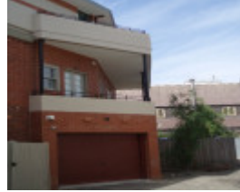
Ferguson Street Residential Precinct, Hobsons Bay Heritage Study 2006 - No. 1 Ferguson St
