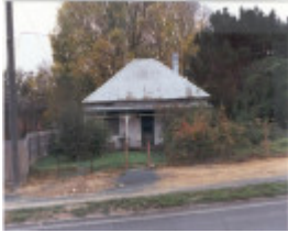
22472 House - 227 Blackburn Road, Doncaster East
