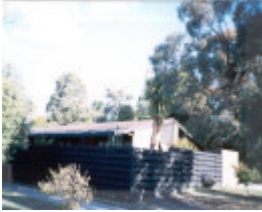
22498 Merchant Builders System House - 1 Exford Place, Donvale (1)
