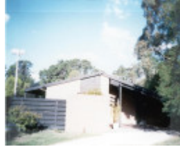
22498 Merchant Builders System House - 1 Exford Place, Donvale (3)
