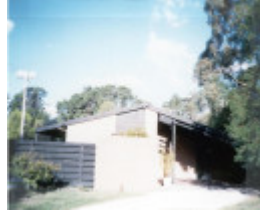
22498 Merchant Builders System House - 1 Exford Place, Donvale (3)
