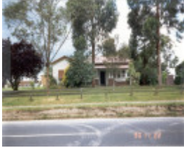
22520 House - 60 Park Road, Donvale
