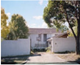
22529 House - 13 Bryson Grove, Lower Templestowe (1)
