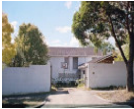
22529 House - 13 Bryson Grove, Lower Templestowe (1)
