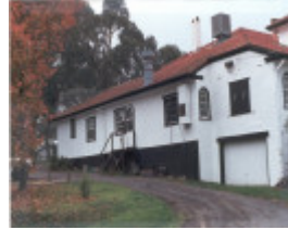
22553 Park Orchards Country Club Chalet - Park Road, park Orcahrds (2)
