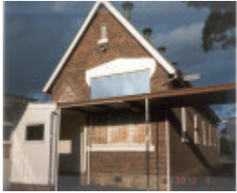
22560 Templestowe Primary School - 1-9 Anderson Street, Templestowe
