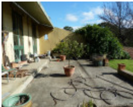
Milking shed floor and west wall - 29 Edwin Road, Templestowe
