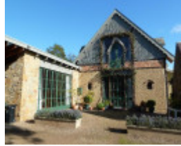
Barn east facade - 29 Edwin Road, Templestowe
