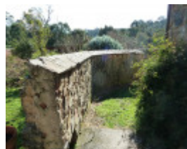
Milking yard wall east side - 29 Edwin Road, Templestowe
