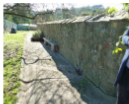
Milking yard wall west side - 29 Edwin Road, Templestowe
