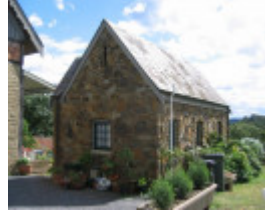
22573 Former Dairy - 29 Edwin Road, Templestowe
