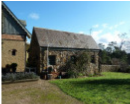
Former dairy - 29 Edwin Road, Templestowe
