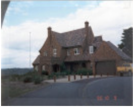
22575 Westerfolds Manor - Fitzsimons Lane, Templestowe
