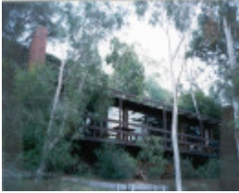
22594 House - 1 Dellas Avenue (Cnr. McLachlan Street), Templestowe
