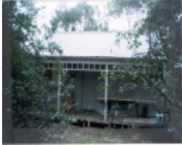
22598 Thyme Cottage - 29-31 Monckton Road, Templestowe
