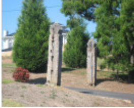
22599 Monckton Gate Posts - 6 Monckton Road, Templestowe
