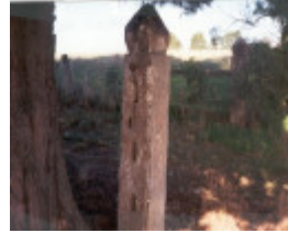
22599 Monckton Gate Posts - 6 Monckton Road, Templestowe (3)
