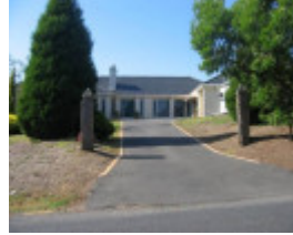
22599 Monckton Gate Posts - 6 Monckton Road, Templestowe (2)
