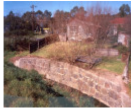
22605 Ruffey's Creek Miners Wall & Swimming Pool Wall - rear 61 Parker Street, Templestowe
