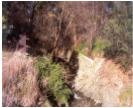
22605 Miners Wall & Swimming Pool Wall - 108 Parker Street (rear), Templestowe (A)
