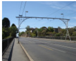
22610 Victoria street bridge richmond march07 ac gantries
