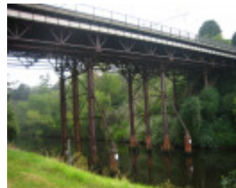
22610 Victoria street bridge richmond feb07 renee 2
