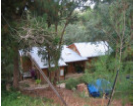
22632 House - 151 Brackenbury Street, Warrandyte (2)
