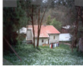
22632 House - 151 Brackenbury Street, Warrandyte
