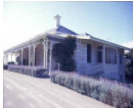
h01899 the anchorage nepean hwy sorrento side view she project 2003
