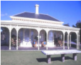
h01899 the anchorage nepean hwy sorrento front exterior she project 2003
