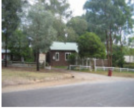
22660 St Stephens Anglican Church - 5-7 Stiggant Street, Warrandyte (1)
