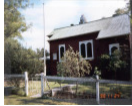
22660 St Stephens Anglican Church - 5-7 Stiggant Street, Warrandyte (2)
