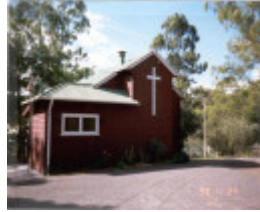
22660 St Stephens Anglican Church - 5-7 Stiggant Street, Warrandyte (3)
