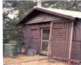
22667 Blacksmiths Building - Tills Drive, Warrandyte (2)
