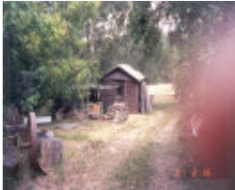
22667 Blacksmiths Building - Tills Drive, Warrandyte (1)
